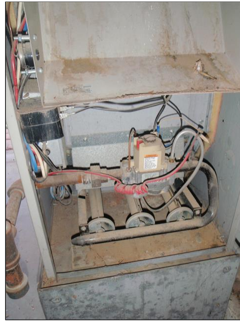
4.13 UNIT HEATER/FURNACE Item 2(Picture)
