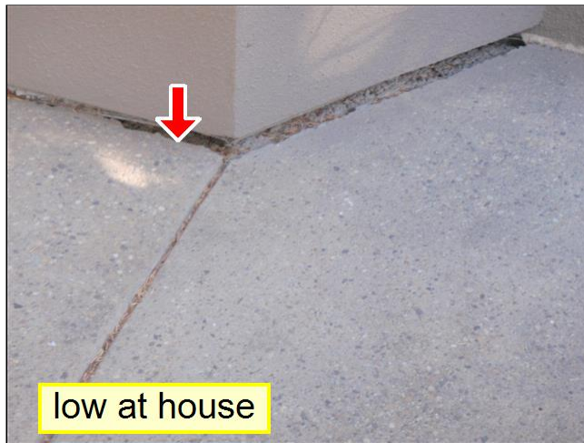
3.1 WALKWAYS Item 1(Picture)
