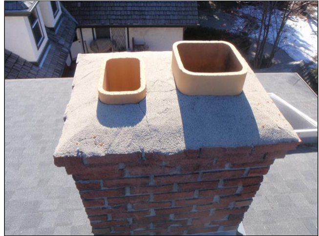
1.1 CHIMNEYS / VENTS #1 Item 1(Picture)
