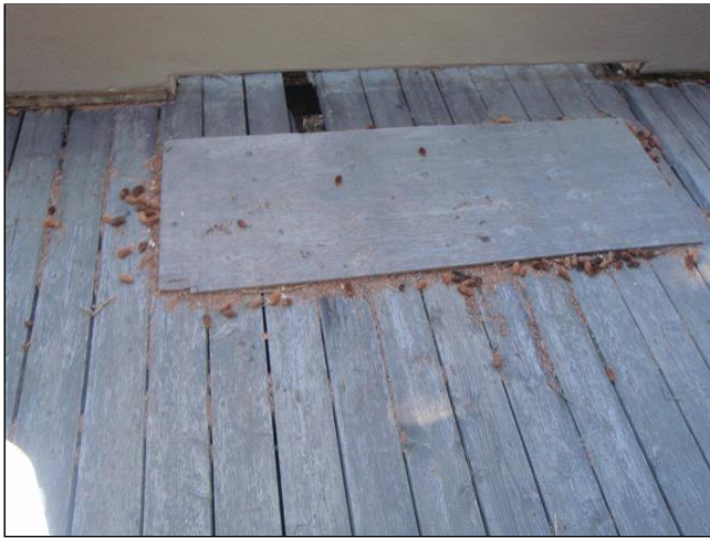
2.6 PORCH(ES) / DECK(S) #2 Item 2(Picture)
