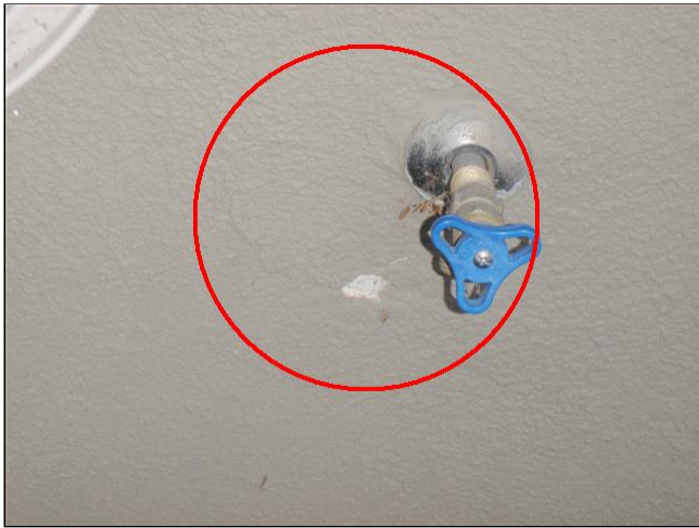
2.0 SIDING #1 Item 3(Picture)
