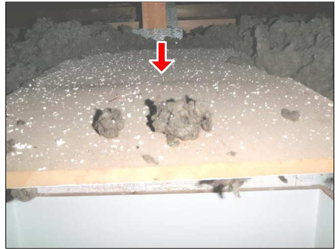
5.5 ATTIC HATCH Item 3(Picture)
