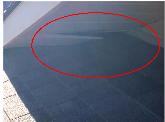
1.10 FASCIA / SOFFITS Item 1(Picture)
