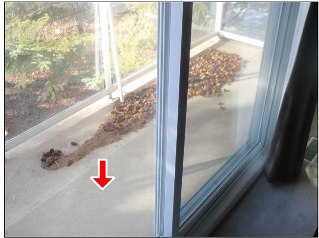
2.7 PORCH(ES) / DECK(S) #3 Item 1(Picture)
