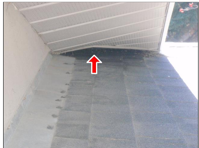
1.10 FASCIA / SOFFITS Item 3(Picture)
