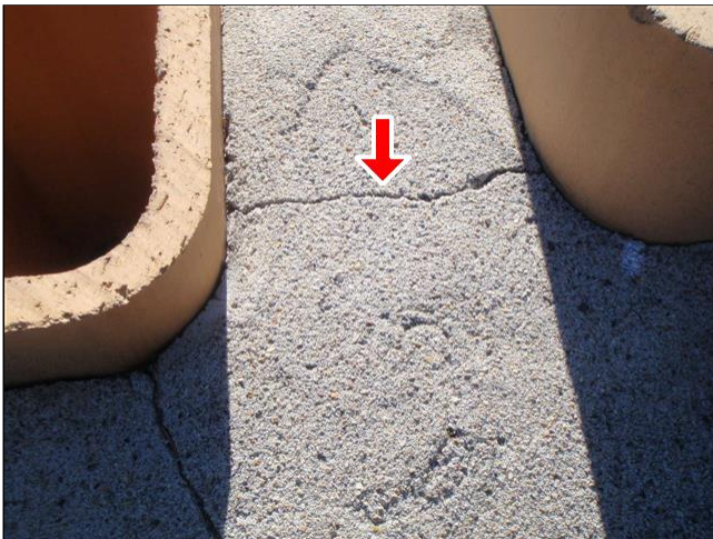
1.1 CHIMNEYS / VENTS #1 Item 2(Picture)
