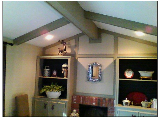
9.1 INTERIOR WALLS (MAIN LEVEL & ABOVE) Item 2(Picture)
