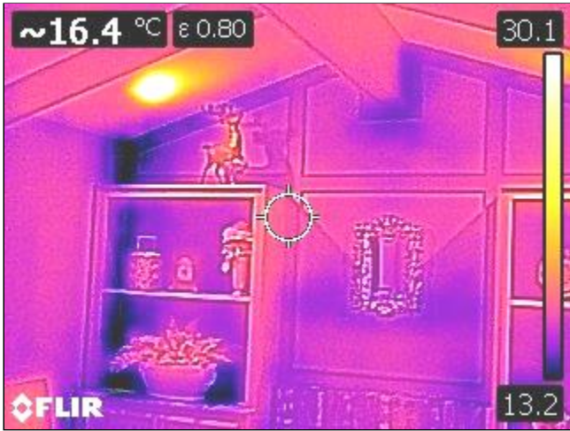
9.1 INTERIOR WALLS (MAIN LEVEL & ABOVE) Item 1(Picture)
