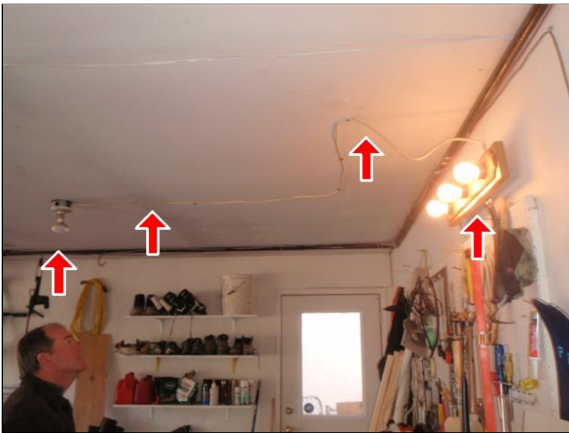
4.11 ELECTRIC / GFCI Item 1(Picture)
