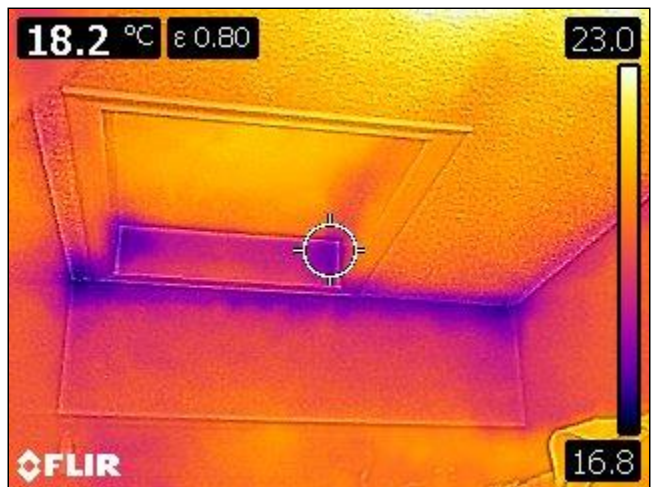
5.5 ATTIC HATCH Item 1(Picture)
