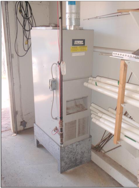
4.13 UNIT HEATER/FURNACE Item 1(Picture)
