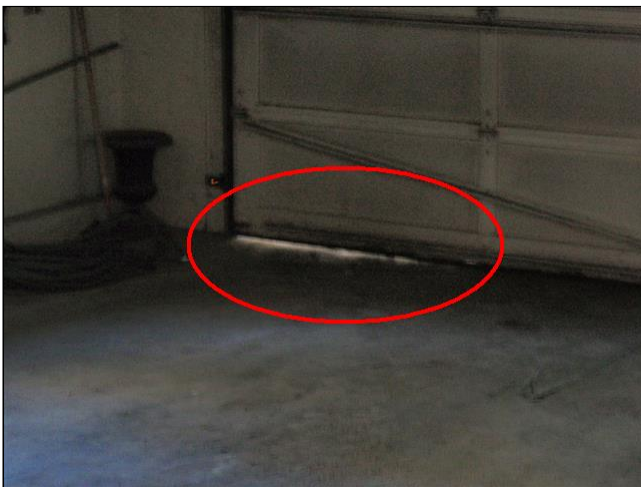
4.9 VEHICLE DOOR(S) Item 1(Picture)
