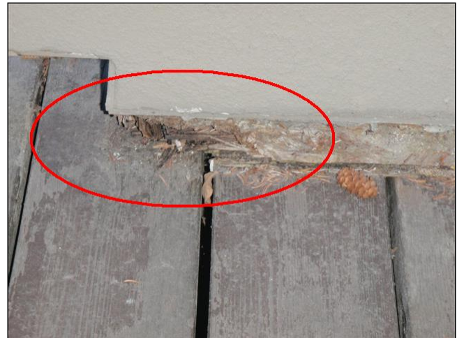
2.6 PORCH(ES) / DECK(S) #2 Item 1(Picture)
