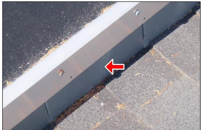
1.5 SKYLIGHT(S) Item 2(Picture)
