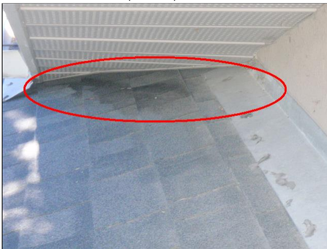
1.10 FASCIA / SOFFITS Item 2(Picture)
