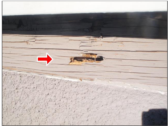
1.2 CHIMNEYS / VENTS #2 Item 1(Picture)
