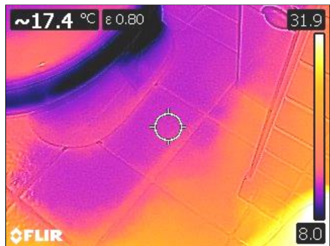
6.1.B TOILET Item 2(Picture)
