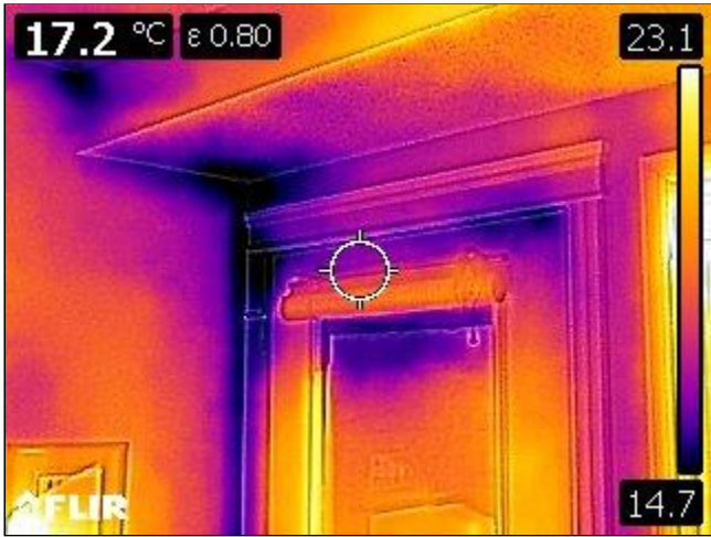
9.1 INTERIOR WALLS (MAIN LEVEL & ABOVE) Item 7(Picture)
