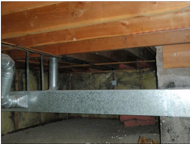
10.3 FLOOR FRAMING Item 1(Picture)
