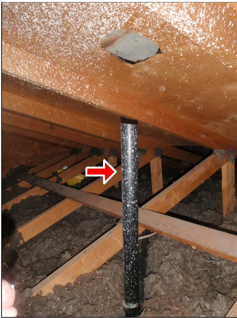
5.4 FLUE(S) Item 1(Picture)
