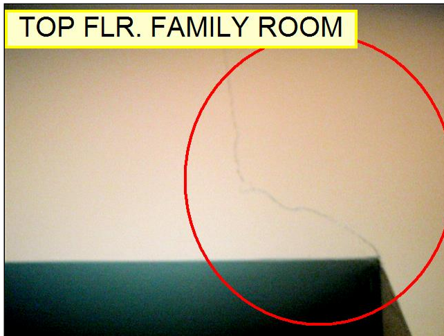
8.1 WALLS Item 1(Picture)
