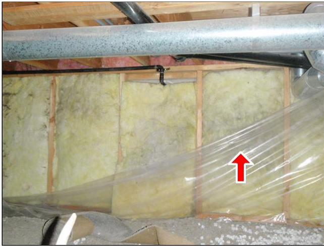
10.0 CRAWL SPACE Item 1(Picture)
