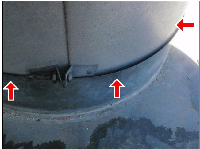
1.2 CHIMNEYS / VENTS #2 Item 3(Picture)
