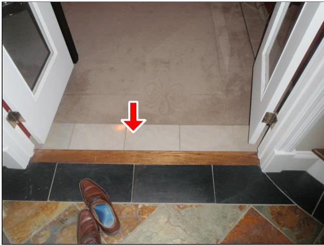
8.6 ROOM DOORS Item 1(Picture)
