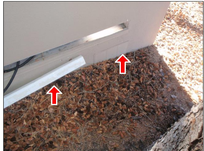
2.0 SIDING #1 Item 2(Picture)
