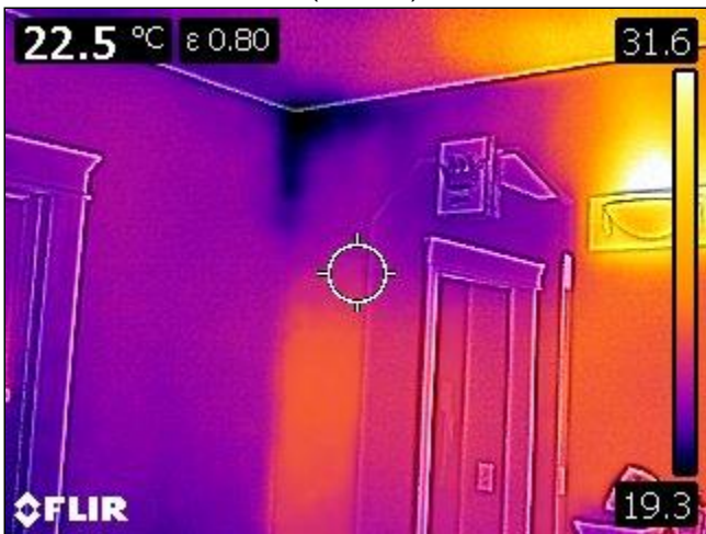
9.1 INTERIOR WALLS (MAIN LEVEL & ABOVE) Item 5(Picture)
