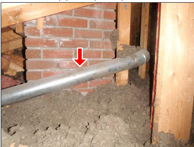
5.4 FLUE(S) Item 3(Picture)
