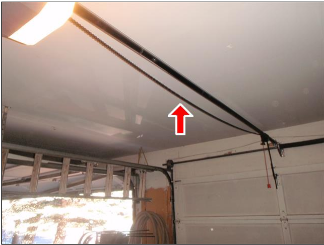
4.10 DOOR OPERATOR(S) Item 2(Picture)
