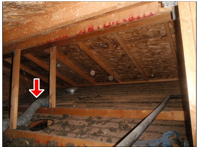
5.4 FLUE(S) Item 2(Picture)
