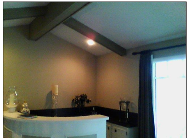
9.1 INTERIOR WALLS (MAIN LEVEL & ABOVE) Item 4(Picture)
