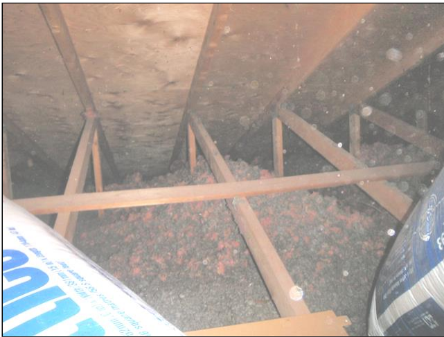
4.5 WALLS / CEILINGS Item 1(Picture)
