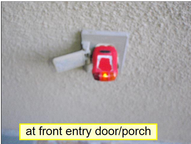
2.10 ELECTRICAL/GFCI Item 1(Picture)
