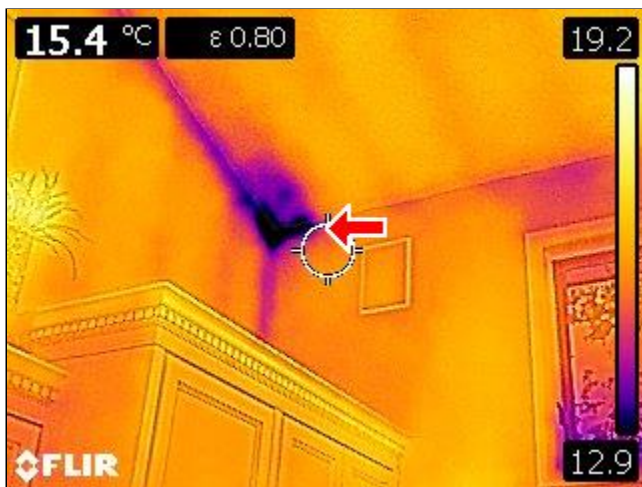
9.0 CEILINGS (MAIN LEVEL & ABOVE) Item 1(Picture)
