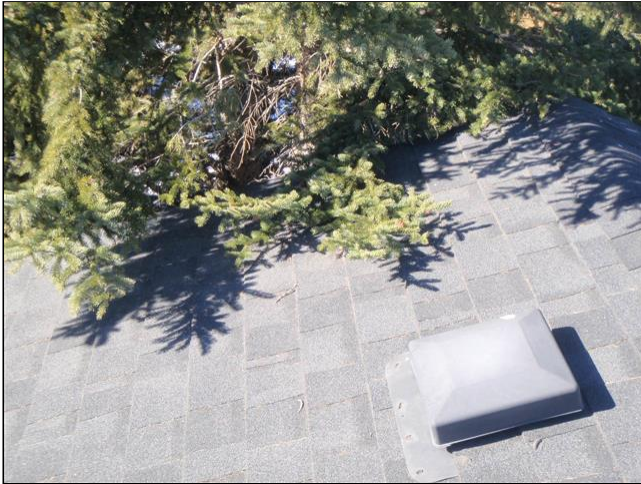
1.0 ROOFING #1 Item 1(Picture)
