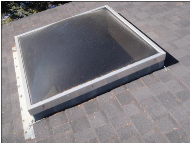
1.5 SKYLIGHT(S) Item 1(Picture)
