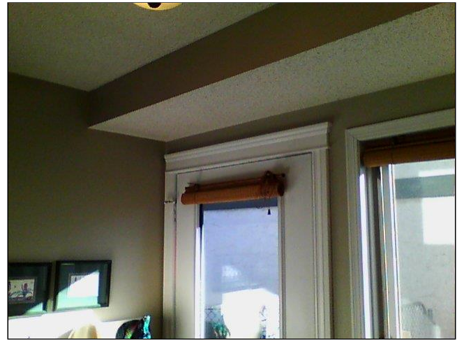
9.1 INTERIOR WALLS (MAIN LEVEL & ABOVE) Item 8(Picture)
