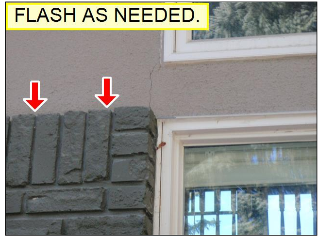
2.1 SIDING #2 Item 1(Picture)
