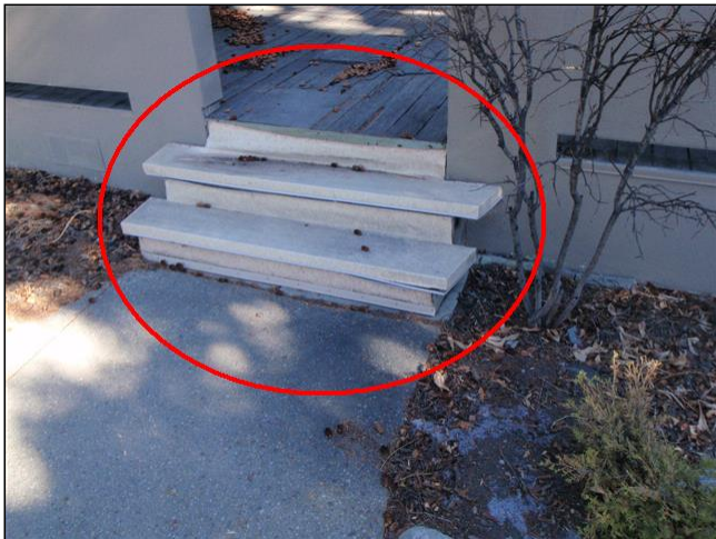
2.4 STAIRS Item 1(Picture)
